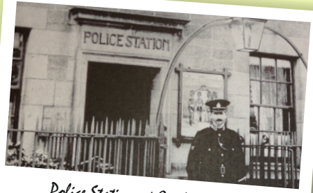
Police Station at Gordon Street
